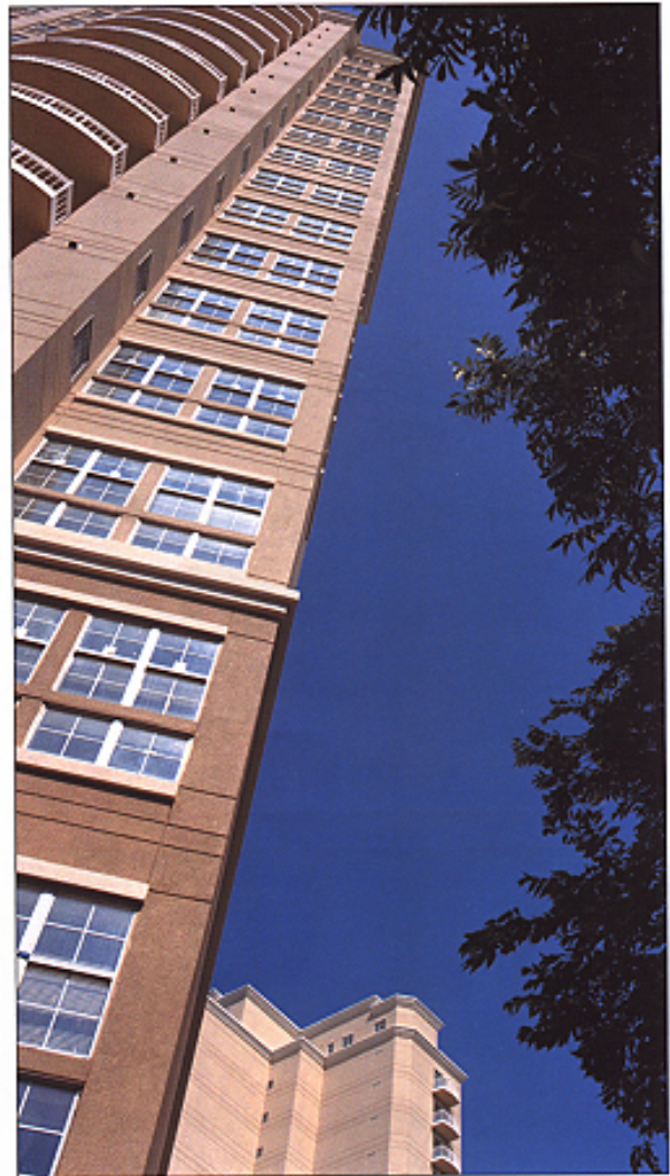
3225 towers over Turtle Creek Blvd.
