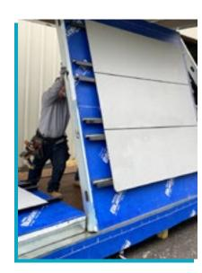
\* Including facade elements such as rainscreen metal panels EIFS etc. into the Pillar EP prefabrication process, adds significant economies of scale. \* Installing the panels is a breeze. Once the units are delivered and distributed to their floor location, the field crew tilts the panel in place over the preinstalled track.
