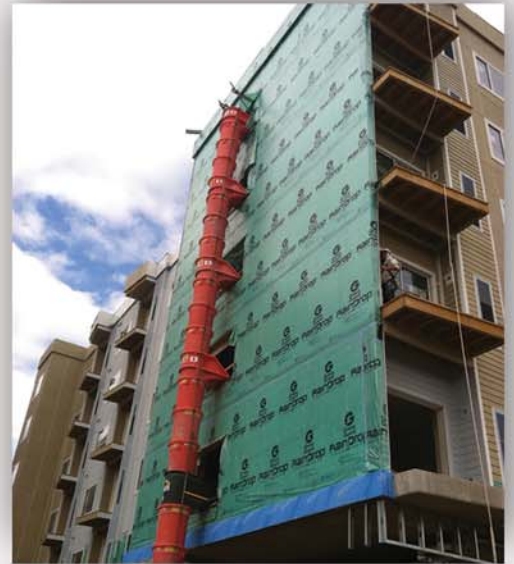
Self adhered membrane behind cement siding Silver Spring MD
