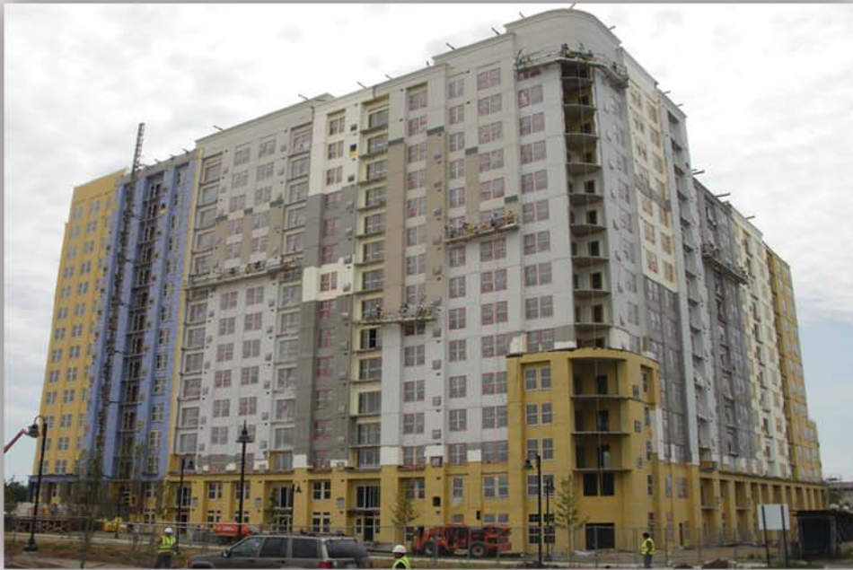
Liquid applied air barrier over exterior sheathing Stamford CT
